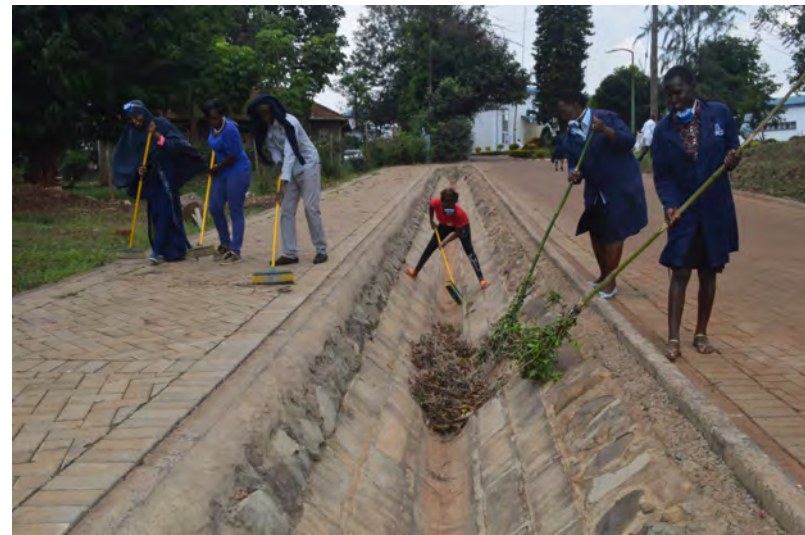
Cleaning of the drainage system
