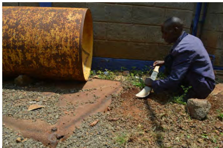
Uprooting weeds around the treatment plant
