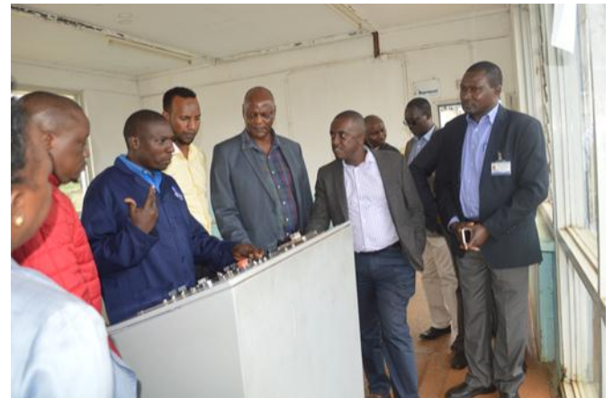
Board Chairman, Mr. Kamba, (5th left) and the Board members listen attentively as staff demonstrates on the technical operations at Ngethu Treatment Works
