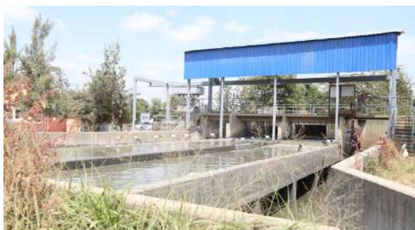
Refurbished section of the Plant
