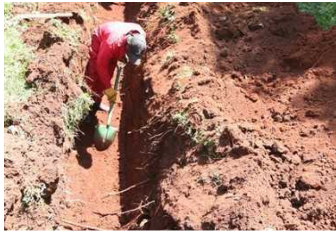
Workers on site digging up the trench
