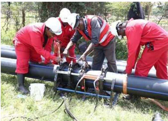
Contractors on site laying the pipes
