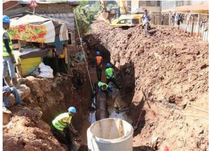
Ongoing rehabilitation of sewer line in Waithaka ward
