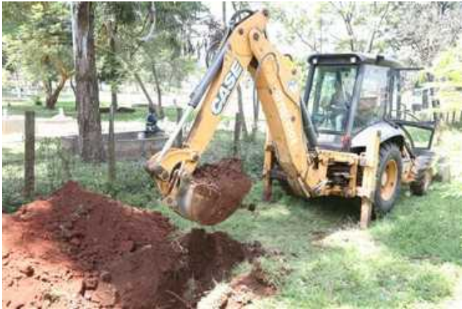
Ongoing excavation works
