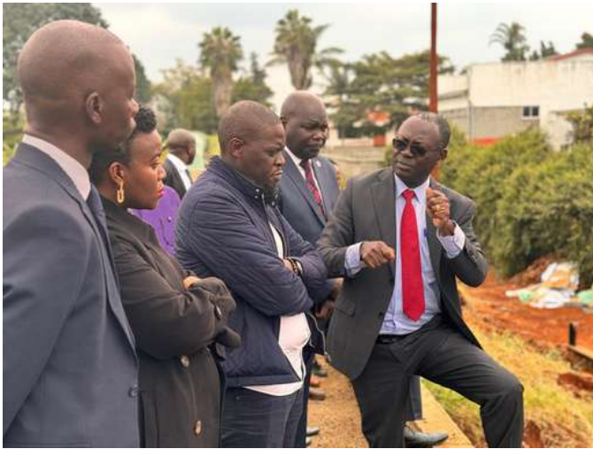
Managing Director, Eng. Nahason Muguna, explains to Nairobi City County Governor, H.E Johnson Sakaja, the technical operations at Gigiri Pumping Station when he toured the facility to inspect the ongoing inlet works in readiness for water from the Northern Collector Tunnel Phase I
