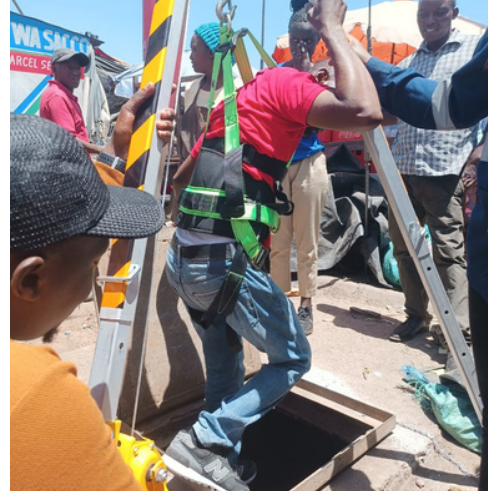
Distribution team being trained on confined entry space using a tripod and winch gear system
