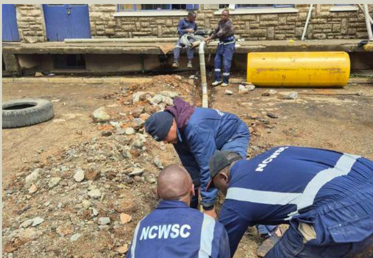
Laying of network cables at Sasumua Treatment Plant
